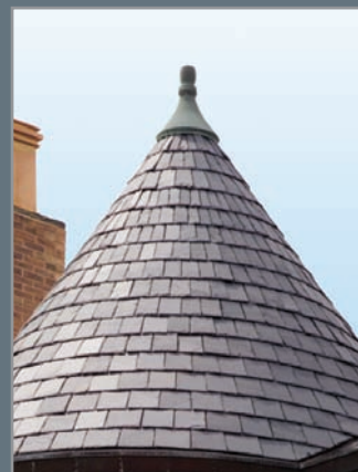
Cone Slate Roof - Dodd Hall, Princeton University
